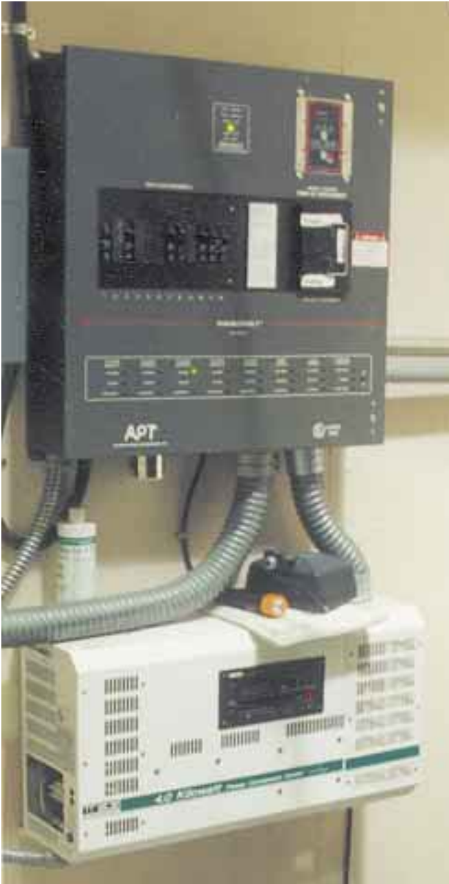
The Ananda Power Center and Trace SW4024 came prewired and were bought used.
