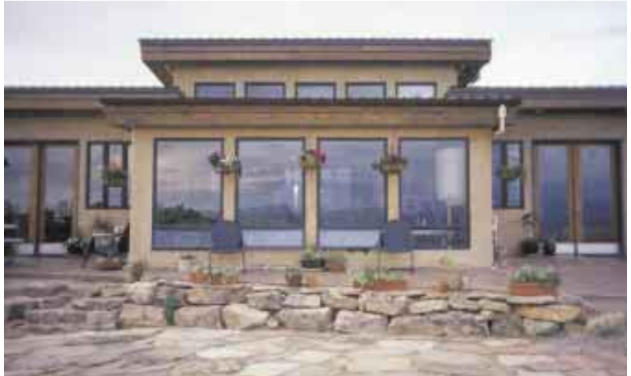
Southern view of the house showing the sunroom, which acts as a double envelope for the living space.
