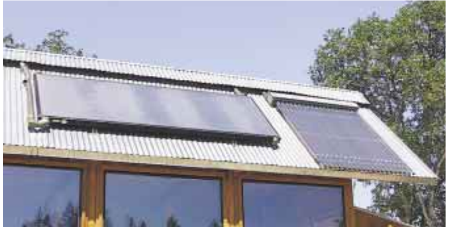
A flat plate (left) and an evacuated tube (right) solar collector.
