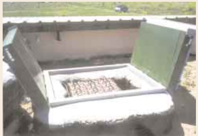
A rammed earth and tire battery box.
