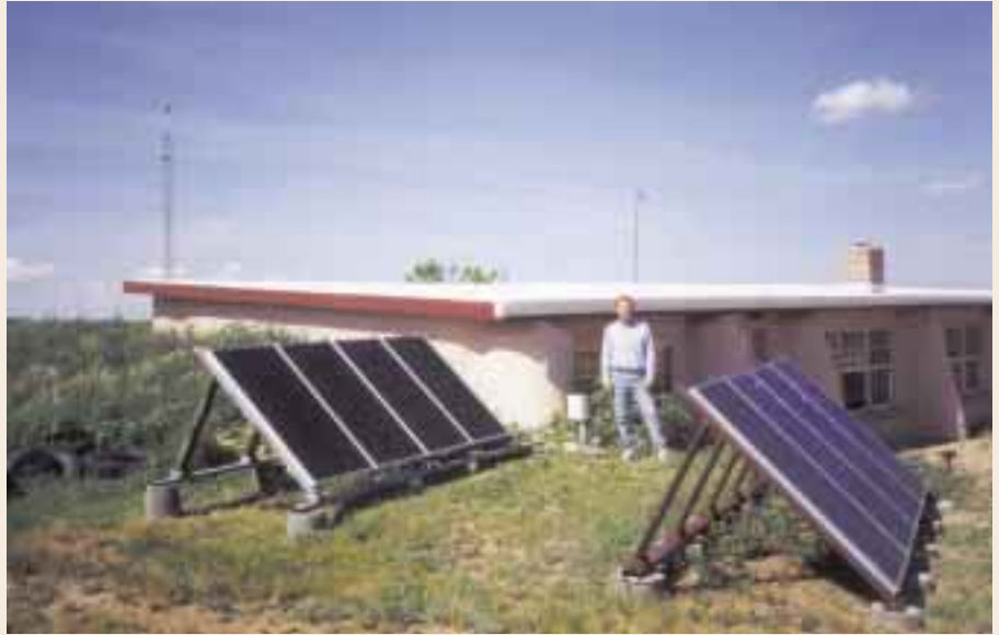
The author with eight Uni-Solar 64 watt photovoltaic modules. Their glassless design makes for hail-proof durability.
