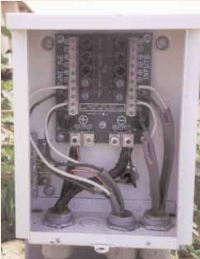
The Trace TCB10 PV combiner box provides fusing for each series string of photovoltaic modules.
