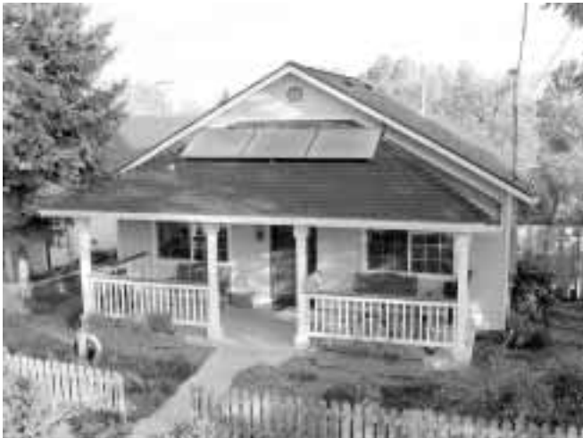
Hot water panels on the front porch roof and the 30 watt PV panel that runs the circulation pump.
