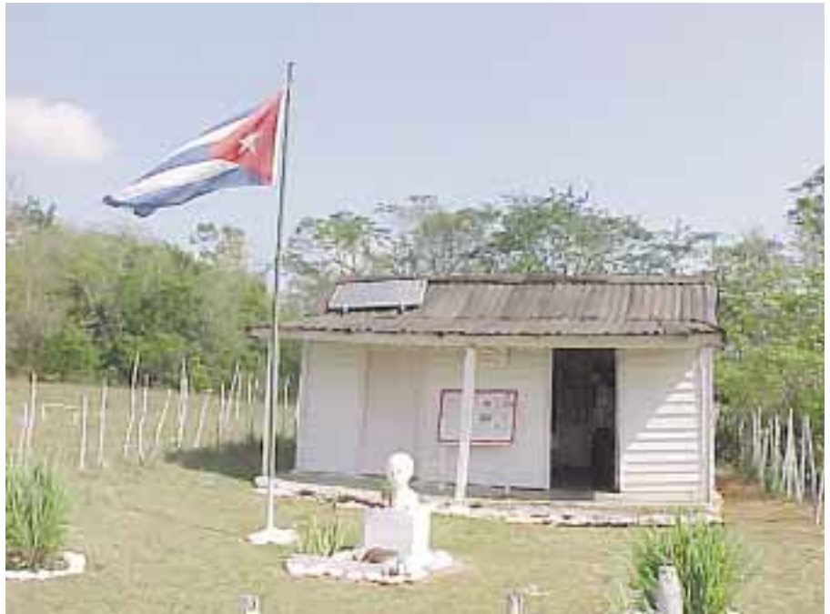
Rural primary school in Pinar del Rio Province.
