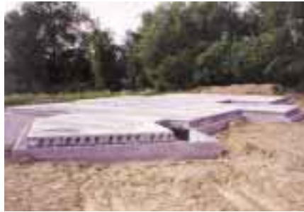
Spancrete forms the main floor decking and offers significant thermal mass.
