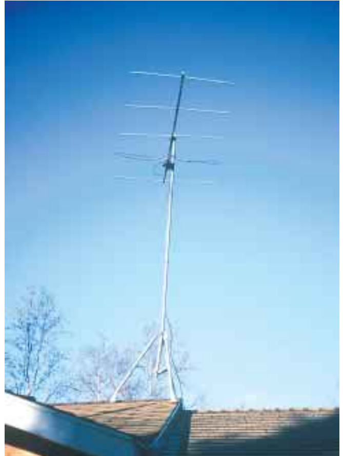
Bill’s homebuilt FM antenna mounted on a recycled TV antenna mast.
