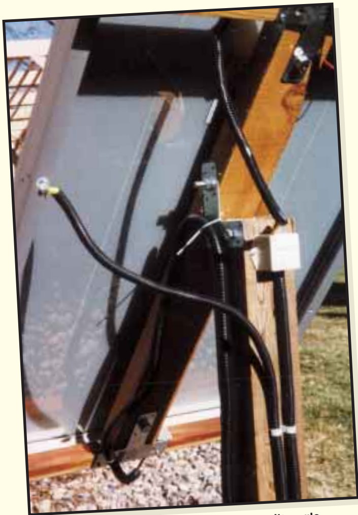
Hamlet's mechanism for adjusting tilt angle Azimuth is adjusted by moving the whole mount.
