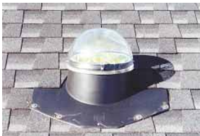
“Solar tube” skylights reduced lighting loads at the inn.
