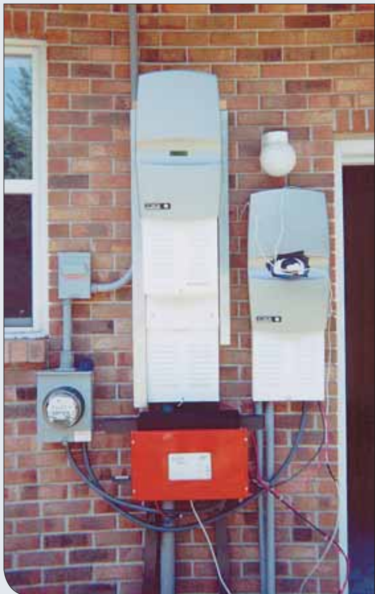
Henry Cutler's wall of inverters includes a Xantrex ST2500 (right), a Xantrex STXR2500 (upper left, mounted on top of one of the original ST2500s), and an SMA SB2500U (lower left).
