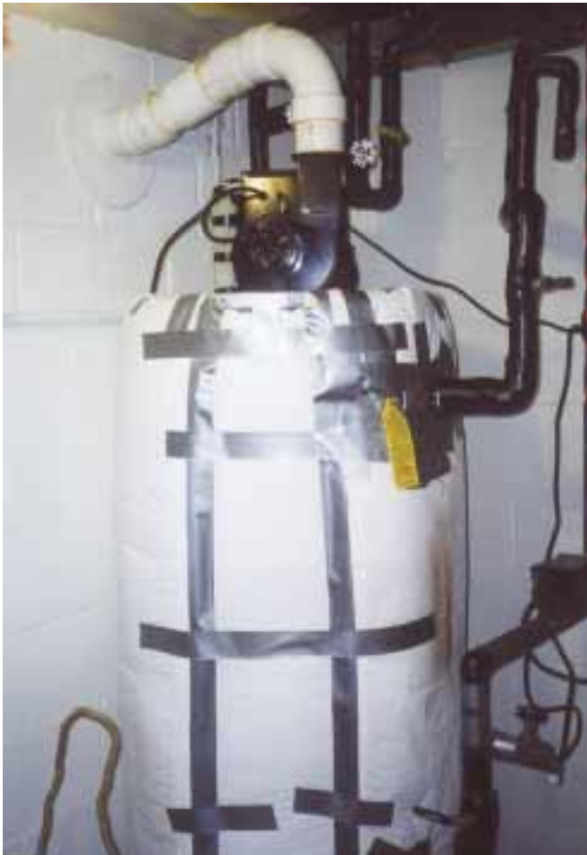
The heavily insulated, backup, natural gas water heater.
