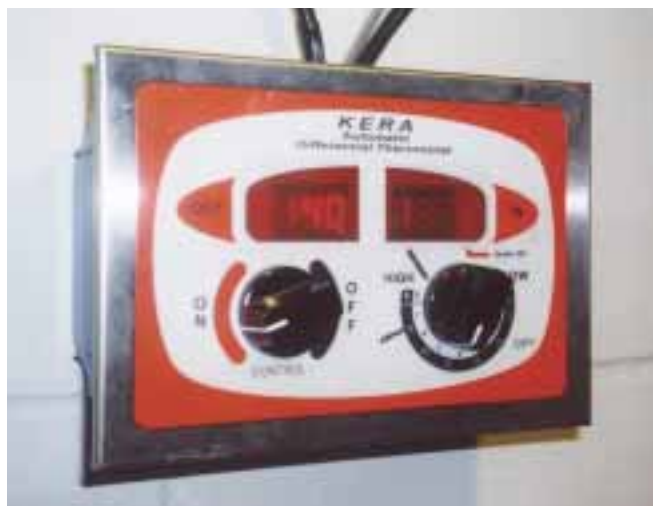
A Kera differential thermostat controls operation.
