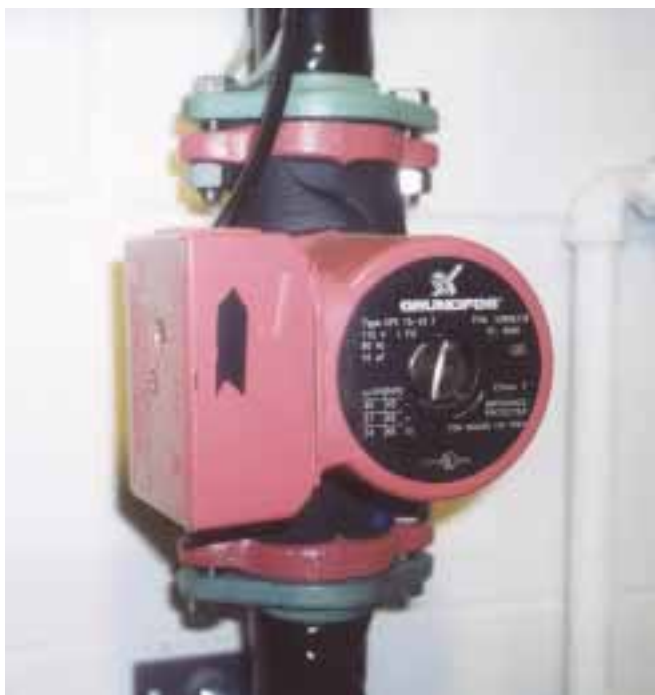
The single, AC powered, Grundfos circulating pump.
