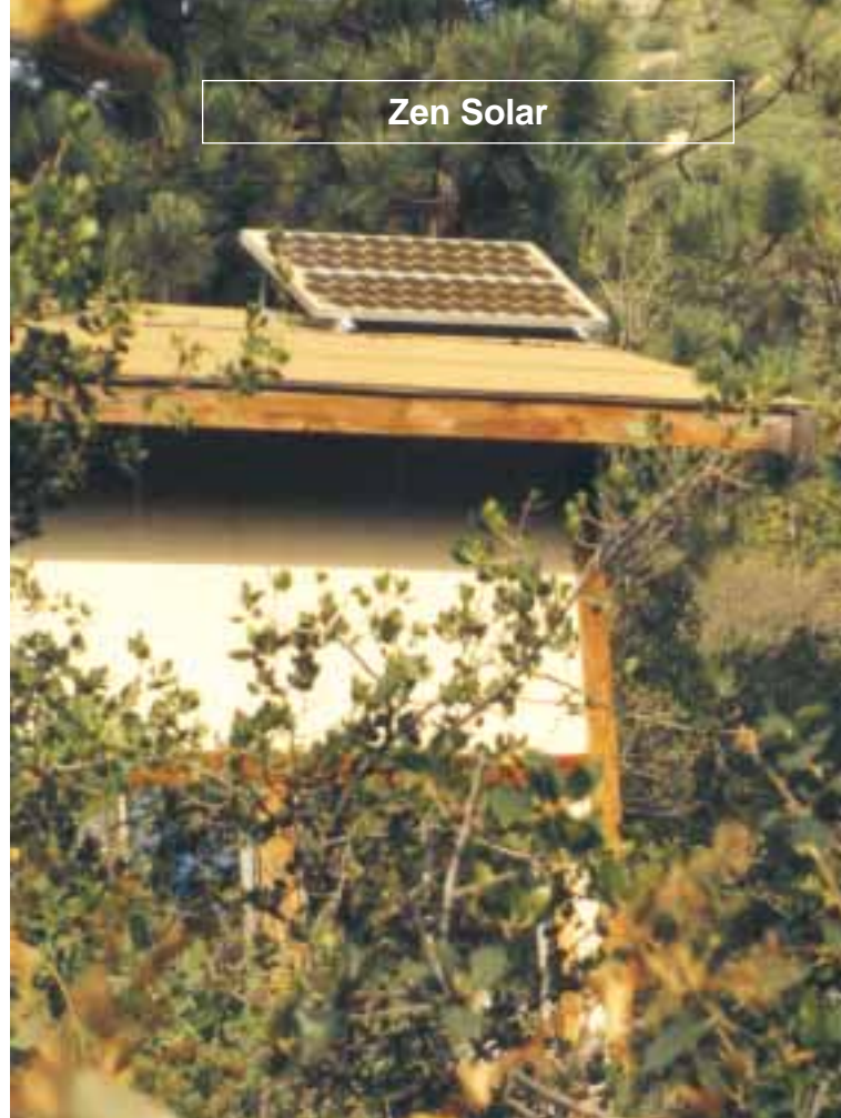
The outlying cabins rely on their own PV systems—a couple of panels, a charge controller, and batteries. The only electrical amenity is 12 volt lighting.
