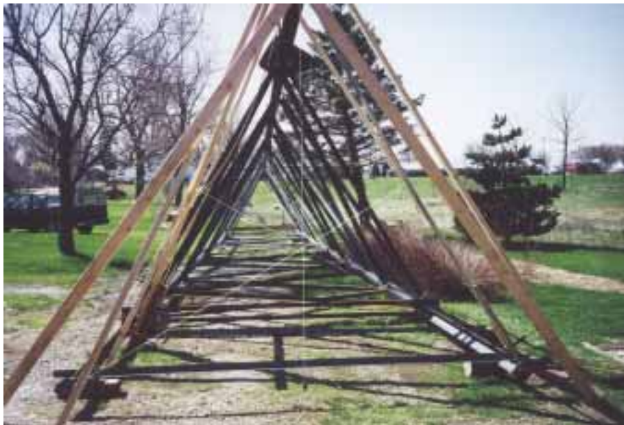
Alignment is crucial for the tower pieces to fit together and to be structurally sound. But a three-legged, tapered tower has no plumb component, so string lines were used to create a center line for reference.
