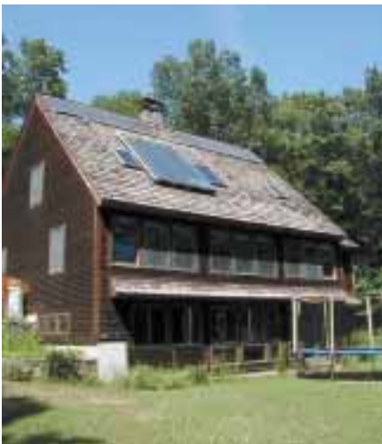
Flush-mounted system.
