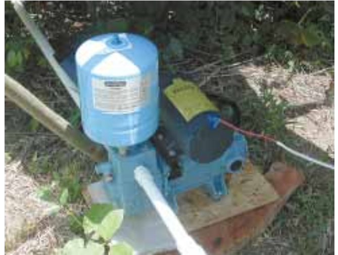
A Dankoff Solar Force piston pump runs efficiently on 24 volts DC from a couple of PV panels.
