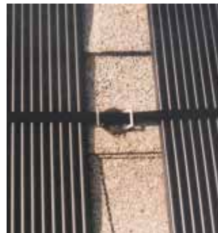
Collector risers are held in place during strong winds by rubber-coated stainless steel straps. The straps are threaded through stainless steel butterfly clips that are screwed to the roof.
