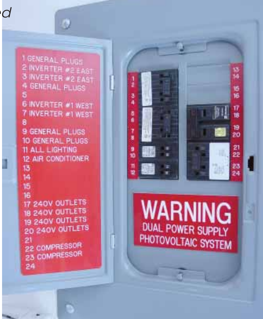
The subpanel that the inverters feed is clearly, safely labeled.
