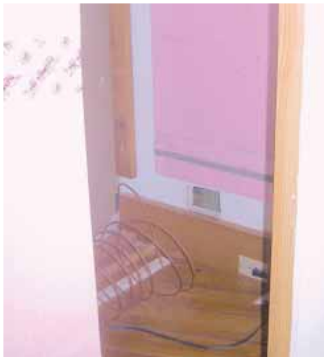
A vent is cut in the wall in the back of the enclosure. The copper coil is the feed for the ice maker.
