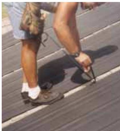
Collector risers are held in place during strong winds by rubber-coated stainless steel straps. The straps are threaded through stainless steel butterfly clips that are screwed to the roof.
