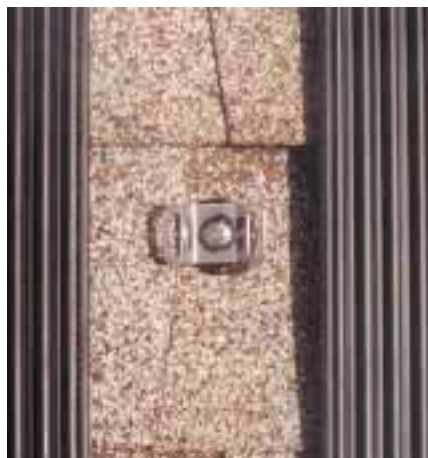
Collector risers are held in place during strong winds by rubber-coated stainless steel straps. The straps are threaded through stainless steel butterfly clips that are screwed to the roof.
