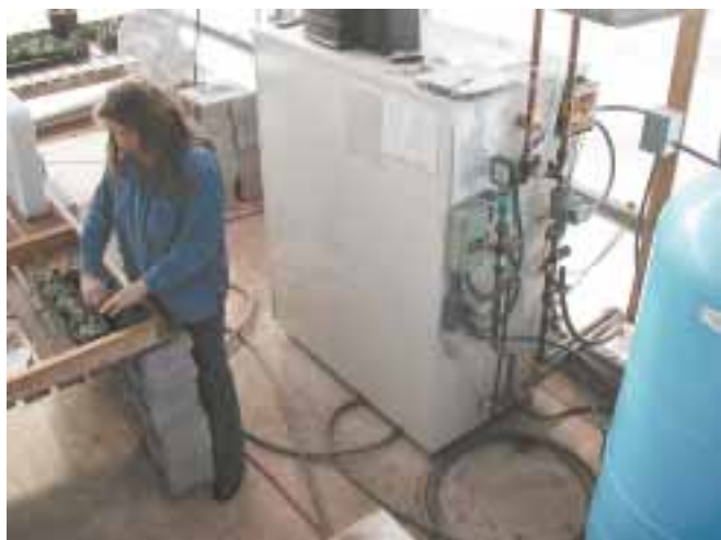
Close-up view of the tank, with the pump, valves, and controls for the solar heating system.
