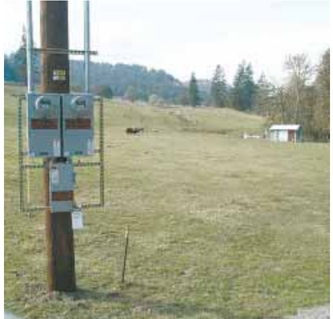
Two KWH meters measure grid energy to the farm and hydro energy to the utility grid.
