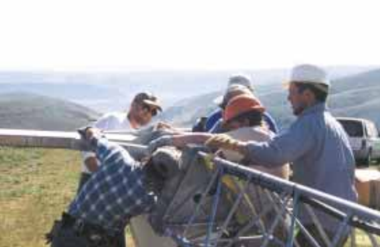
Muscling the Bergey's tail into position.
