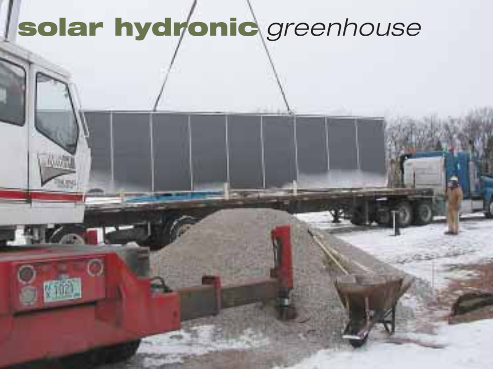
A crane lifts the 2,500 pound, 8 by 40 foot long maxi-collector to its mounts in front of the greenhouse for the Oneida Nation in Wisconsin.
