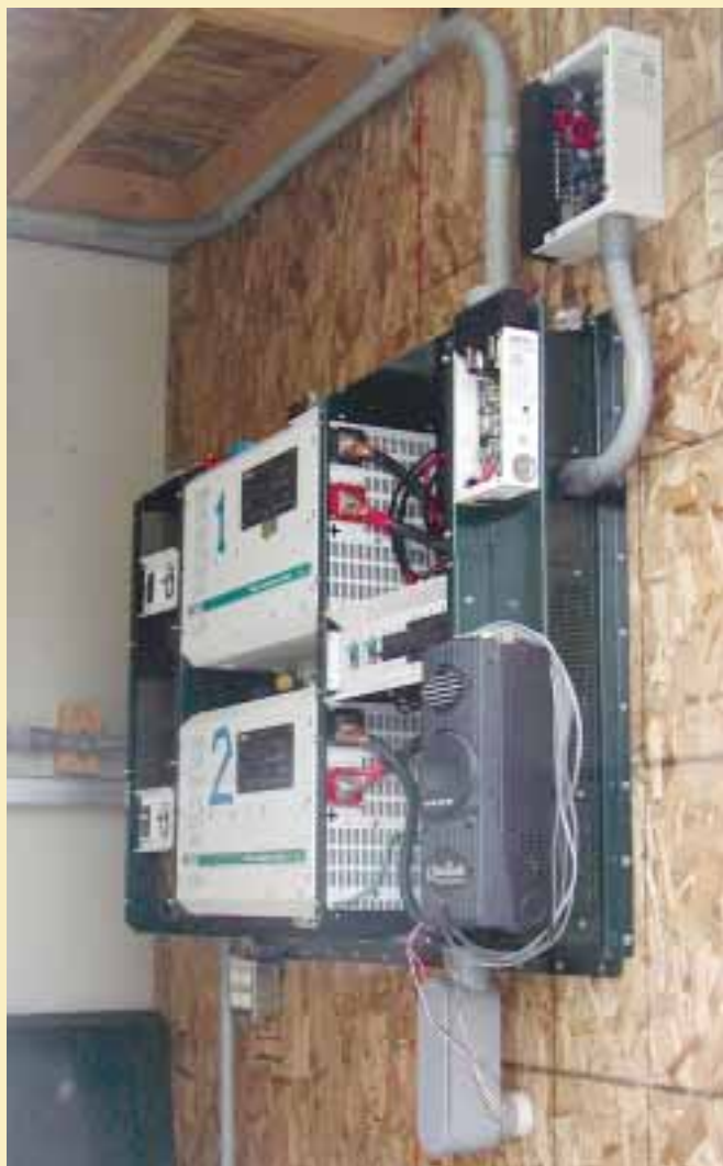
Colorado's power system—two Trace SW5548 inverters, Solar Boost 3048, Trace C40 and Outback MX-60 charge controllers, and Outback power system enclosure.
