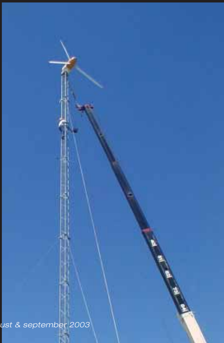
Climbing to unhook the crane.
