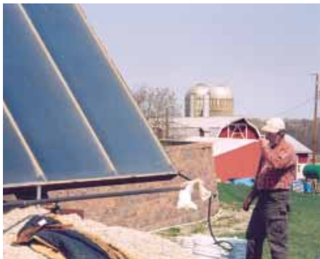
George Zachariasen fills the maxi-collector with the propylene glycol antifreeze mixture.
