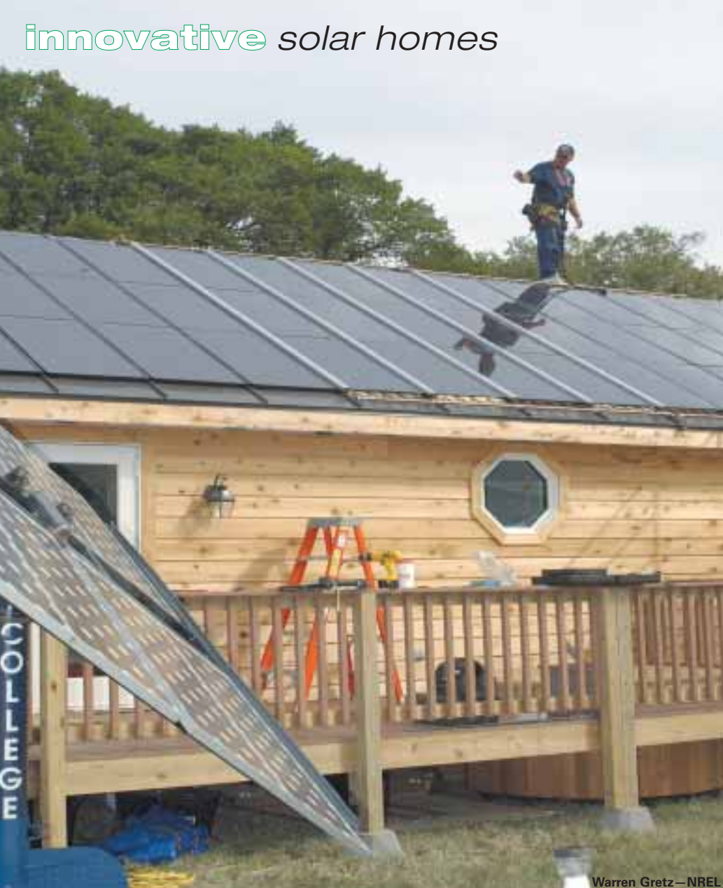
Crowder College's experimental building integrated PV and solar thermal system. Note the exposed plumbing below the PVs on the roof—insulated hot water transfer tubes run below the PVs and heat-absorbing plate.
