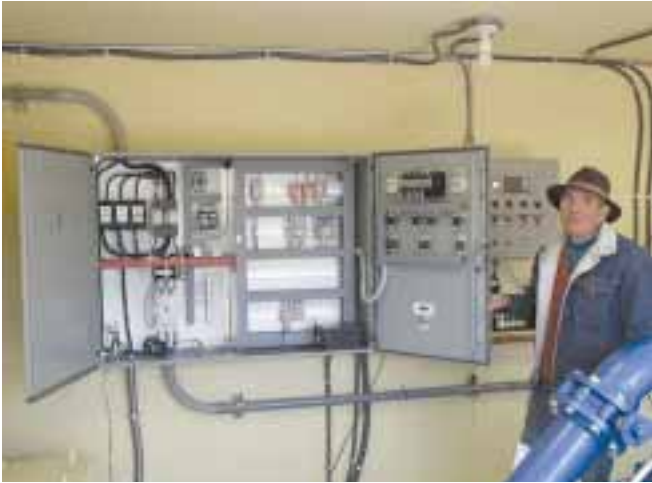
The main contactor enclosure contains the overcurrent protection, manual disconnect, and main relay.
