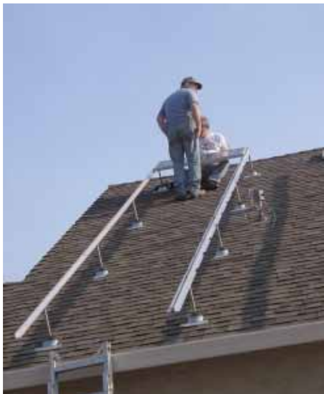
Installing the first PV module.
