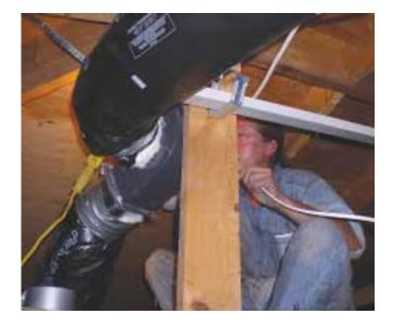
Working in tight quarters—Matt hangs the blower, runs the duct, and then finally wires the system.
