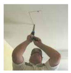
Left: Kris locates and cuts a 6 by 10 inch hole for the hot air register in the ceiling of the living space.
