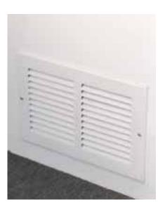
this—the HVAC industry also has a ready-made  $3^{1/4}$  by 10 inch (8.3 x 25 cm) duct that will serve in many instances. No matter what, get the cold air from the floor level of the rooms you wish to heat if you want the system to work.
