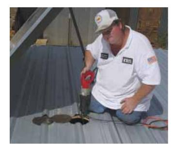
Kris cuts a 9 inch hole, for the 8 inch duct, in exactly the right spot.
