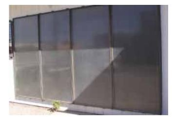
When wall-mounted hot air collectors are feasible, the installation can be very simple.
