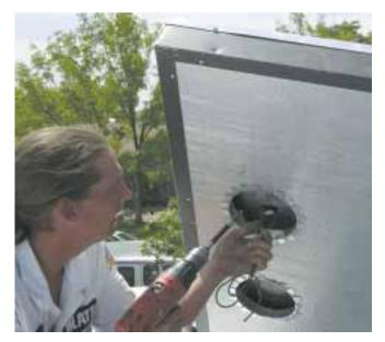
Matt attaches the snap disk in the hot air outlet before connecting the duct. The wires will run between the flexible duct and the rigid duct.
