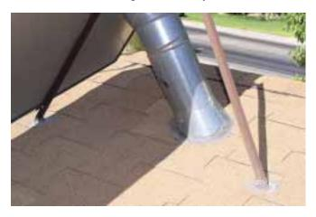
Galvanized duct is used as weatherproofing outside the outer covering of the insulated flex duct, and overlaps the roof jack. Any adjustable elbows for the weatherproofing need to be placed over the insulated flex *before* it is attached to the collector. Straight pieces of duct snap together to connect the elbows to the roof jack, and all of the joints should be sealed with silicone sealant.
