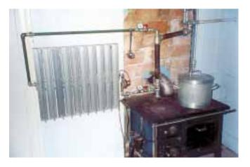
In this nongeothermal application, an oil stove heats water that rises into the thermoelectric generator to power the pump, which sends the heated water to the home's radiators, distributing the heat.
