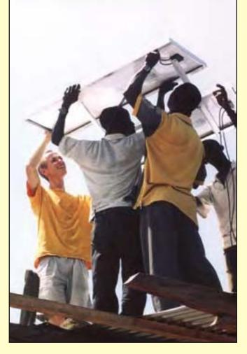
Mounting the panels on the DP&W rack—a 17 foot tall, 2 inch diameter steel pole supports the whole assembly.
