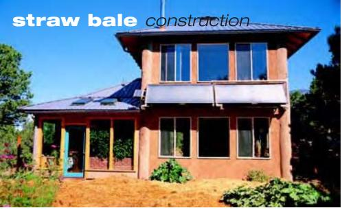
A straw bale wall has ideal qualities for passive solar design. The bales provide insulation for the thermal mass of the interior plaster, which captures the warmth of the winter sun through south-facing windows.
