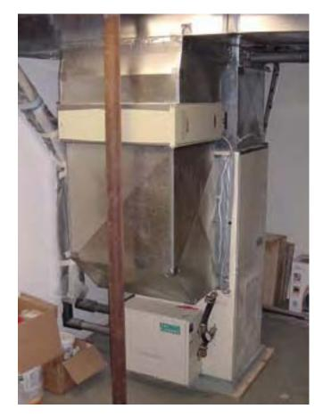
The Econar GeoSouce heat pump adds to the system with heat from 3,000 feet of buried tubing.
