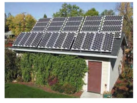
Thirty-two Siemens SR100 photovoltaic panels generate about 85 percent of the Kerr family's electricity.
