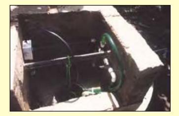
The completed "pump house." The electrical connections are on the left, the plumbing is on the right, and the pump is hanging from the bar in the middle.
