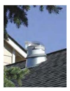
Sun Pipes transmit sunlight directly into the house, offsetting daytime lighting loads. at least 34 phantom and always-on devices that draw a combined minimum of 100 watts 24/7. It works out to be 876 KWH per year, or 15 percent of my annual load.
