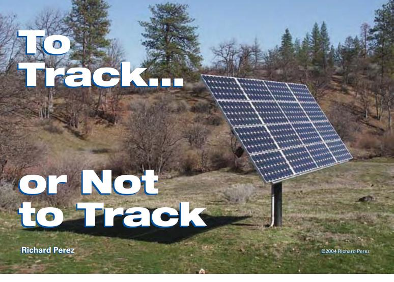
A 1,360 watt PV array on a Wattsun dual-axis tracker follows the sun all day, like a big silicon flower, maximizing solar output.
