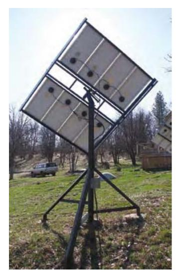
No motors or sensitive electronics on the back of the Zomeworks trackers—simplicity is reliability.
