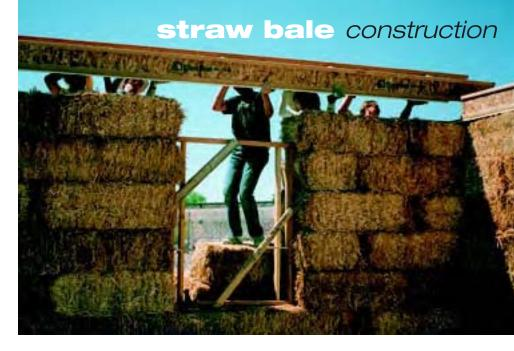
In load-bearing construction, a rigid "top plate" or "bond beam" is placed atop the straw bale walls, joined at the corners and secured to the foundation. This beam allows the weight of the roof to bear equally on all four structural bale walls.
