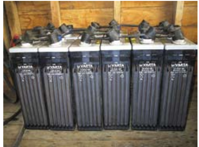
Proper charging, discharging, and maintenance kept these six-year-old batteries in like-new condition.
