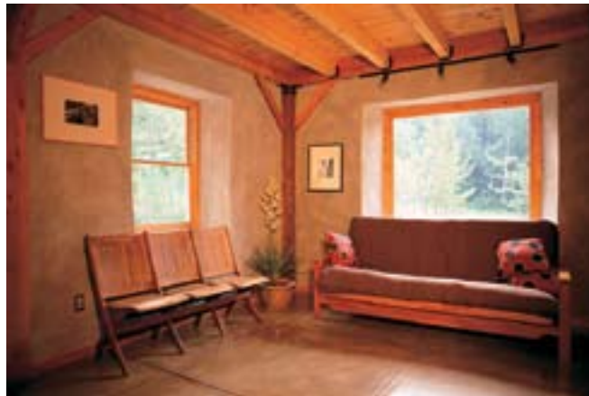
In a post-and-beam house, beams can be exposed on the interior, as shown in this Charlemont, Massachusetts, home.
