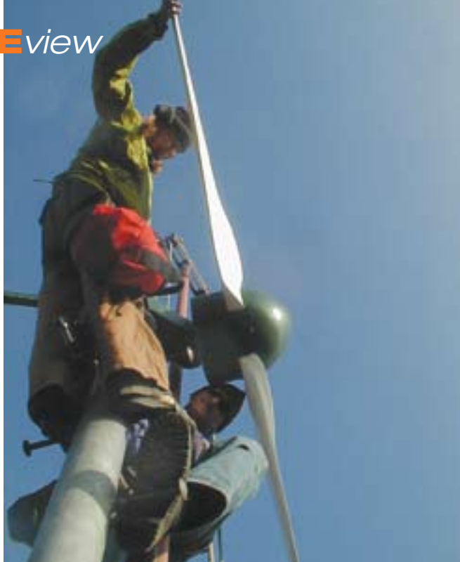
SEI students Nicole Lavick and Eric Youngren finishing the installation of an AWP 3.6 wind generator during a workshop.
