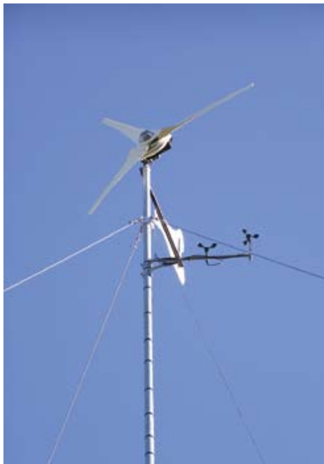
Fully installed turbine. The two anemometers supply wind data, which is accessible at the tower base and inside the power room.
