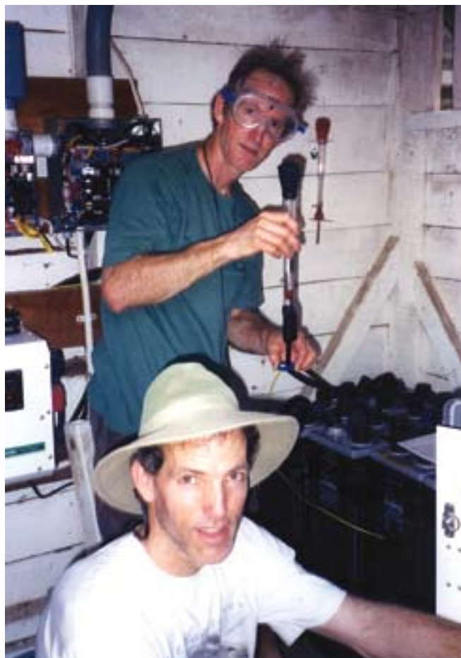
Elliot and Jeff Burch (bottom) check the specific gravity of each cell.
