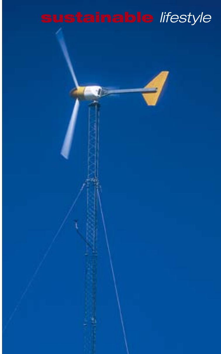
Inn Serendipity's grid-intertied, hybrid electric system features a 10 KW Bergey wind turbine on a guyed, lattice tower.
