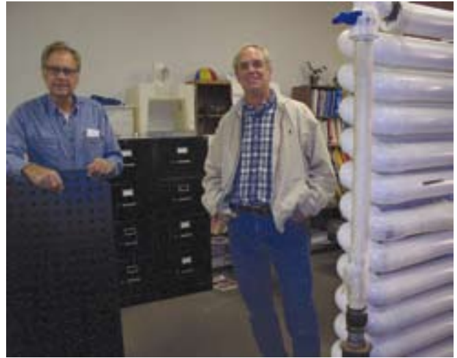
The author and Dave Harrison next to the storage/radiator that heats and cools their offices. The storage pipes also serve as a divider for the two offices.
