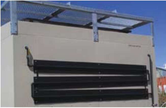
The south wall of a cool cell electronics room that Zomeworks manufactures with the Double Play cooling technology. This doesn't need much radiator surface area since it is designed to keep the room under 100°F.
