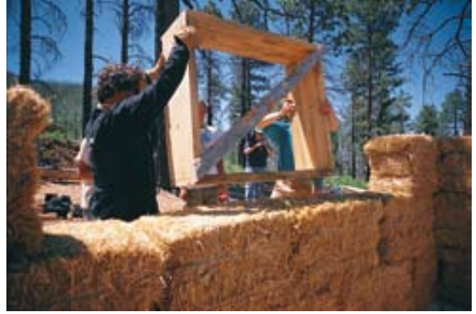
In load-bearing walls, the window "rough buck" is inserted into the bale wall as it goes up.
