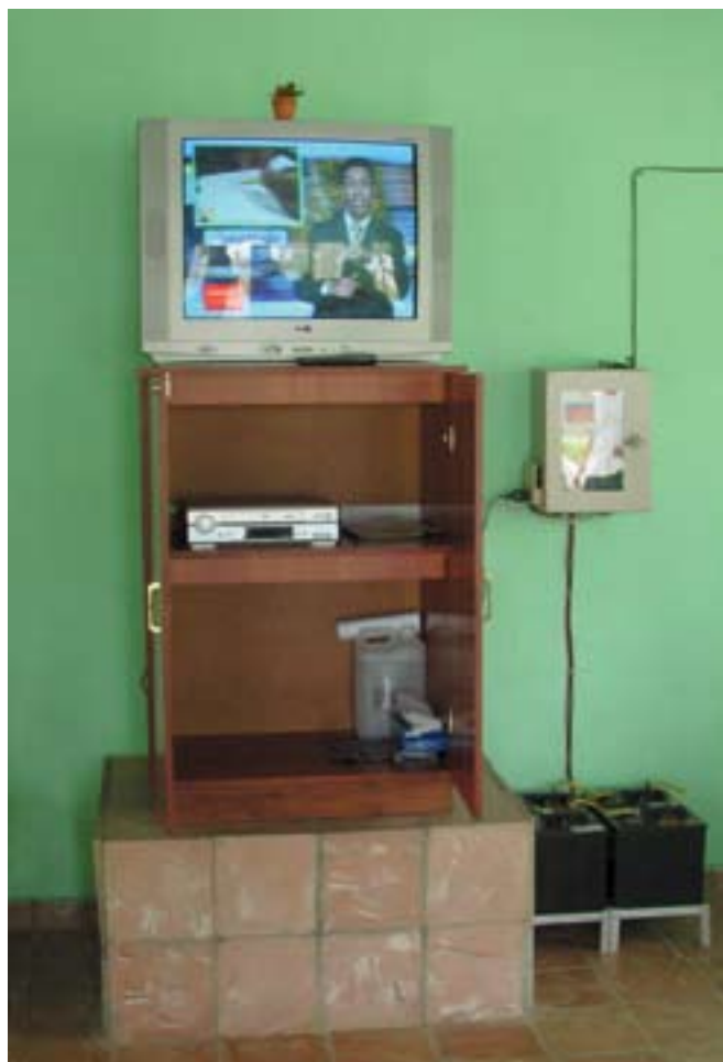
Some of the standard TV sala equipment—TV, inverter, controller, batteries, and VCR.
