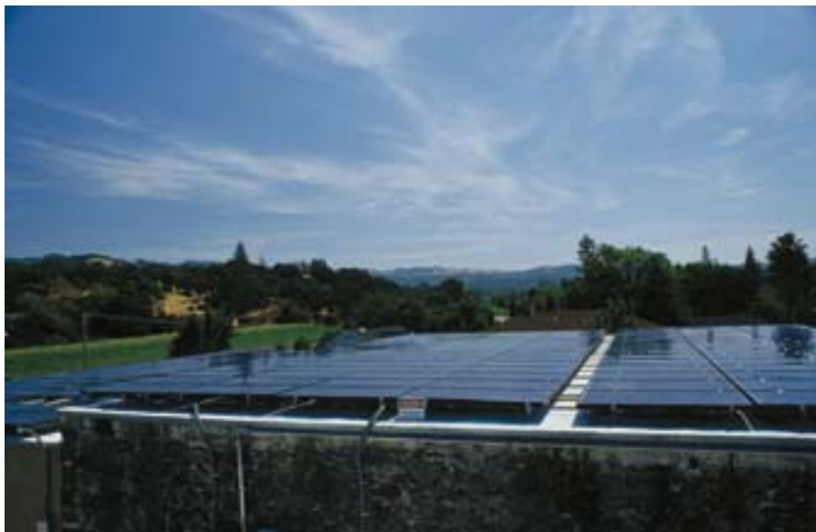
A portion of the 234 BP photovoltaic modules that make up the 30 KW system.
