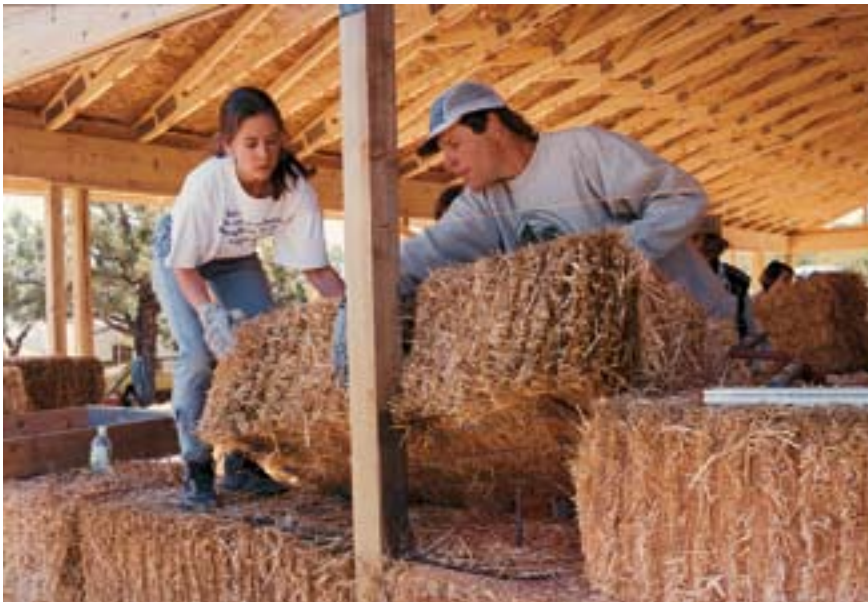
Bales can be notched around posts, or the posts can be left exposed on the interior or exterior.
