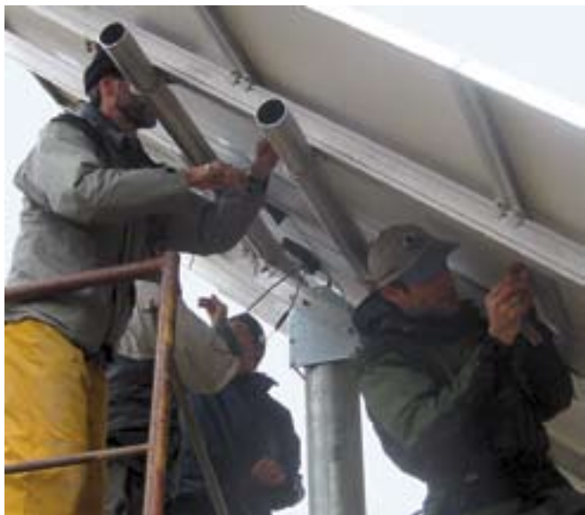
SEI students Larry Owens (left) and Tom Brenton fastening PV modules to the top-of-pole rack.
