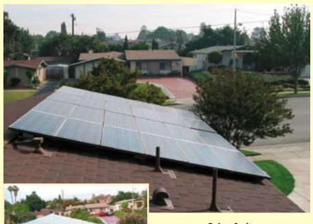
Before & after the inset photo shows the author's experiment to increase the array's efficiency by allowing more airflow under the panels.
