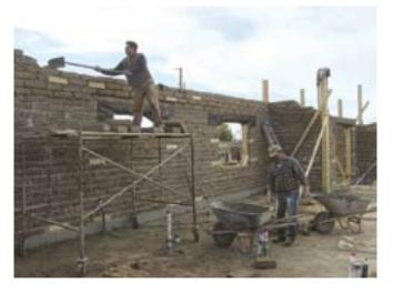
Adobe Mud Throw 2: There goes the mortar onto the wall. Note the speed leads outlining the corners of the walls.
