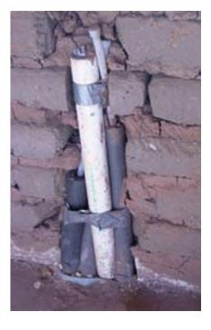
Water lines and a drain line are in place to service the bathroom sink. Adobes and mortar easily fit around the pipes.
