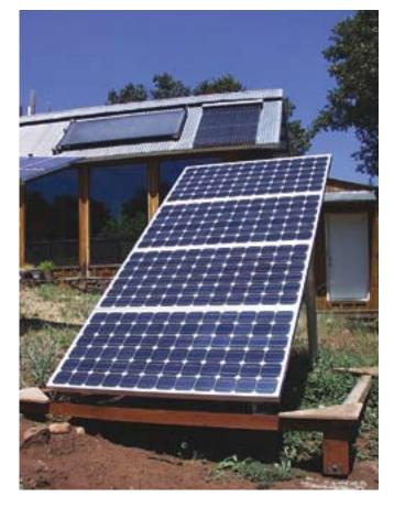
The new PV array—four Sharp, 185-watt modules running at 48 VDC.
