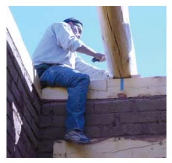
The original code called for 4-inch (10 cm) thick bond beams. It was raised to 6 inches (15 cm), since 4-inch beams are hard to do in concrete. The 4-inch wood bond beam has more tensile strength than the concrete, and is more than adequate for those in nonpermit areas.
