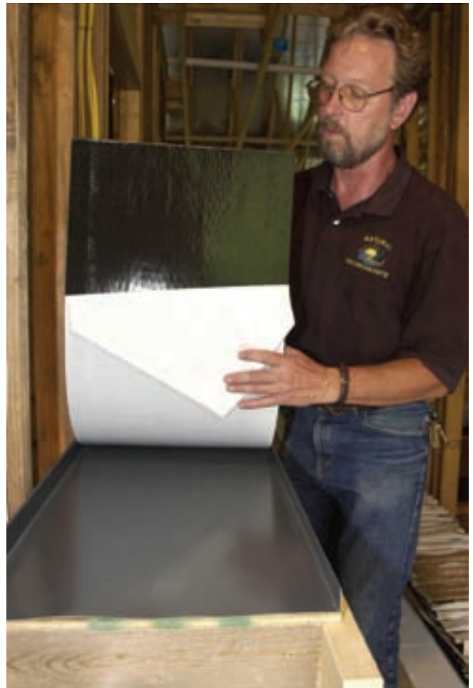
Peeling the backing from the end of a Uni-Solar laminate before adhering it to the metal roofing.
