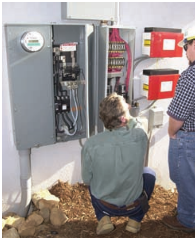
The service entrance showing utility service, array combiner/disconnect, and Sunny Boy inverters.
