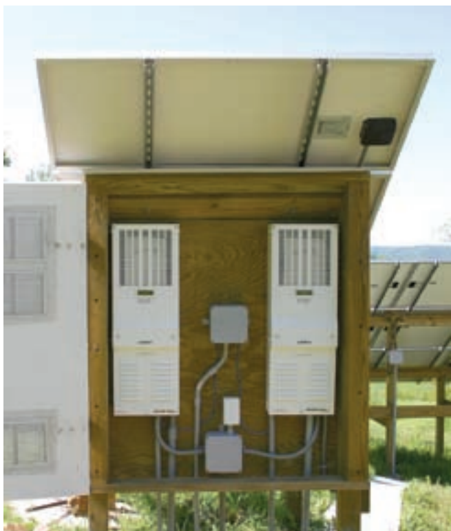
The two Xantrex SunTie inverters in their custom cabinet send the output from the PV panels to the house and utility grid.
