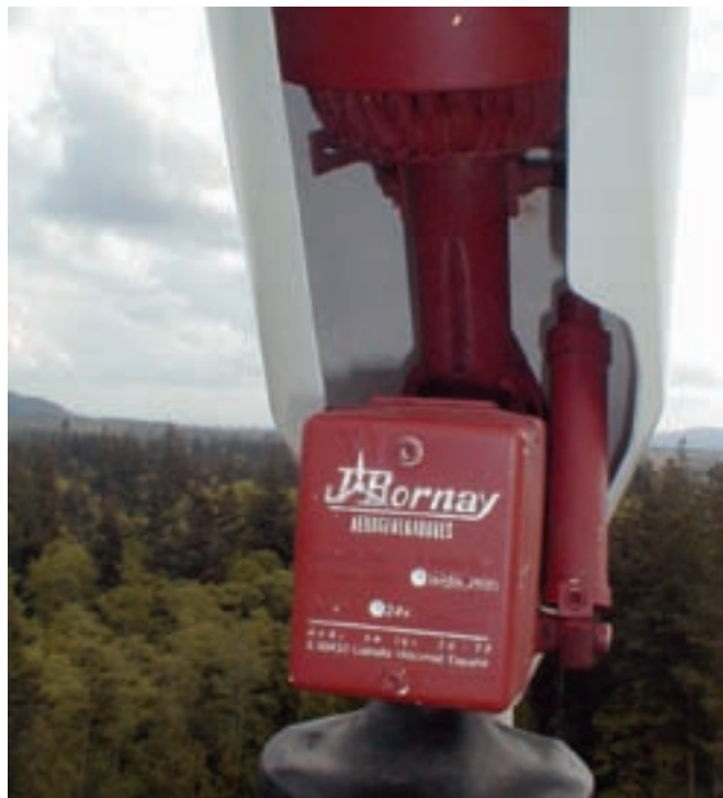
Bornay Inclined 1500 generator and shock absorber in governing position (tilted back).
