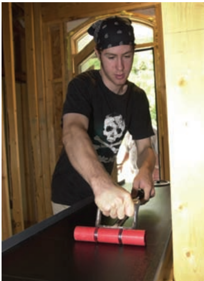
Rolling the PV laminates to ensure complete adhesion.
