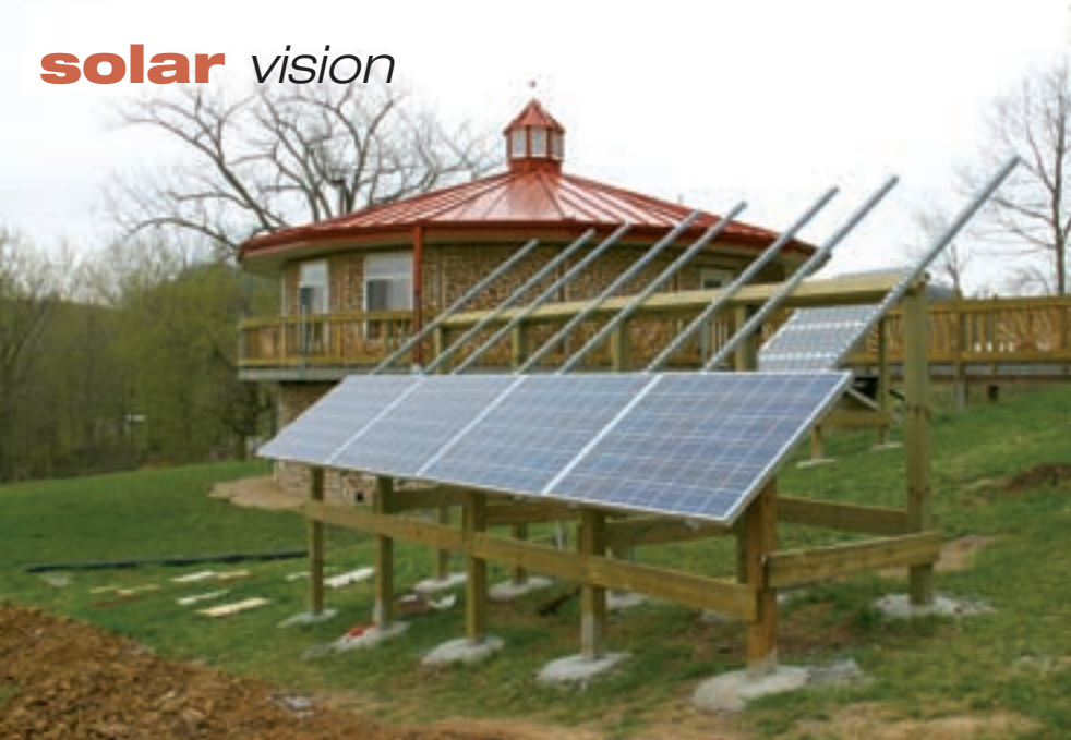
Alan built the PV array mounts himself using pressure-treated lumber and Unistrut rack. They are not adjustable, but set at an angle that maximizes annual production.
