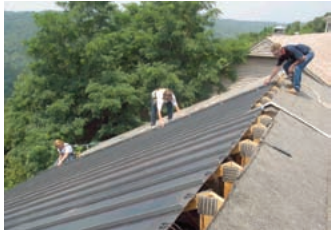
Installing the roof panels.
