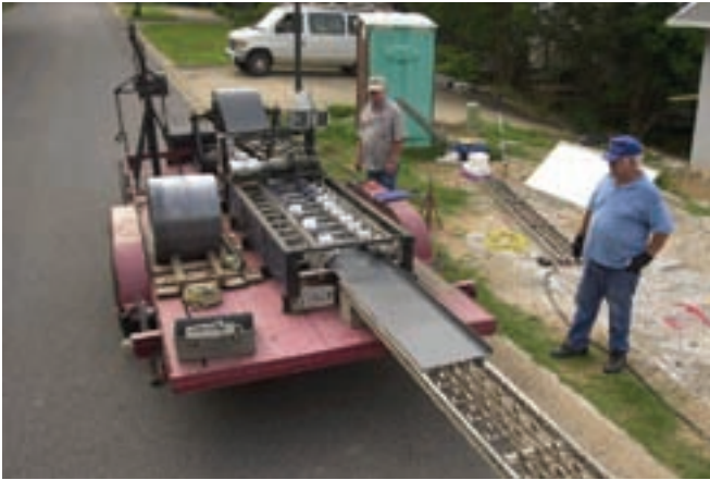
Making the roof panels on site.
