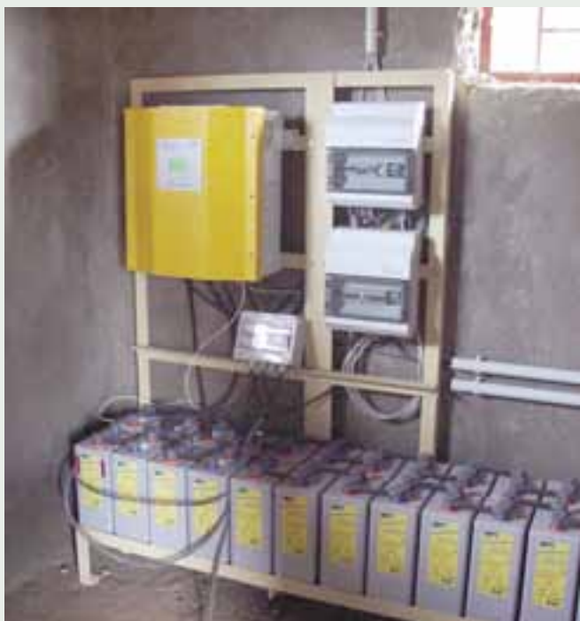
The SMA Sunny Island inverter, battery bank, generator connection box, and two AC distribution boxes.
