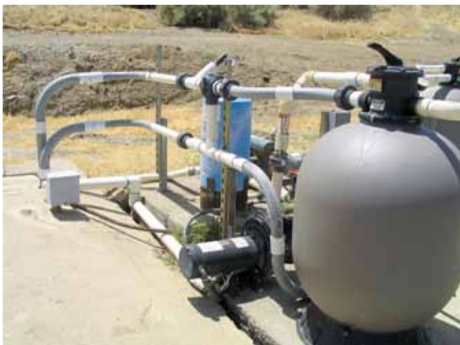
The modified plumbing sends the output of the circulation pump to a three-way valve, through the lower header of the heat exchanger, out the top header, through a ball valve, and back to the filter and chlorinator.
