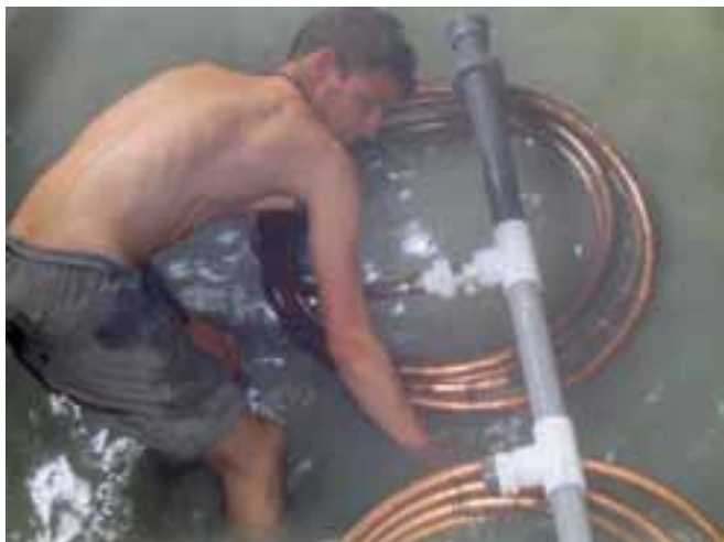
Steve Bain positions three of the heat exchanger coils on the cradle in the partially emptied spring tank. The two final coils were then lowered into the tank and connected to the preassembled ones.
