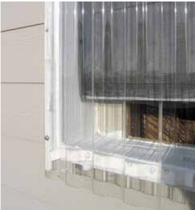
A close view of the lower sill, lower vent, left end's vertical glazing supports, and screen absorber. "Wiggle" closure strips secured to the sill plates help seal the glazing panels.
