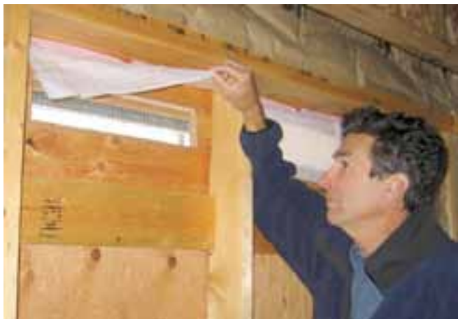
The author inspects the thin plastic flapper valve that prevents reverse airflow and helps keep heat inside the building.
