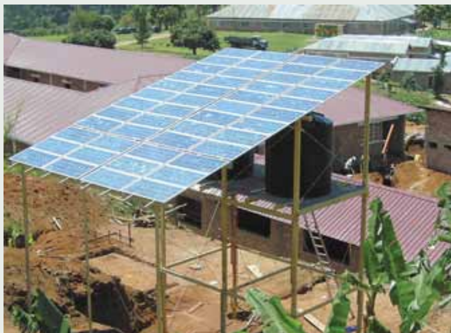
A view of the completed PV installation above the large school compound. An AC mini grid allows optimal placement of system components without the proximity restrictions inherent in DC-coupled systems.
