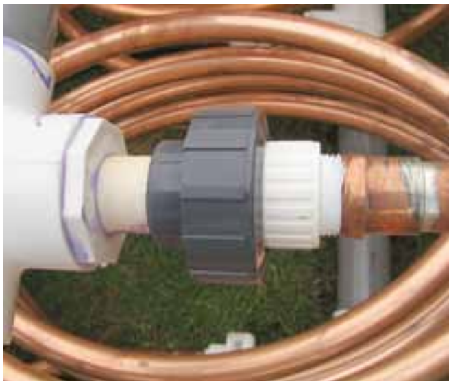
Connection to the manifold required a 2-inch tee, a reducer, a short PVC nipple, the union, and a PVC-to-copper adapter that was soldered to the end of a coil.
