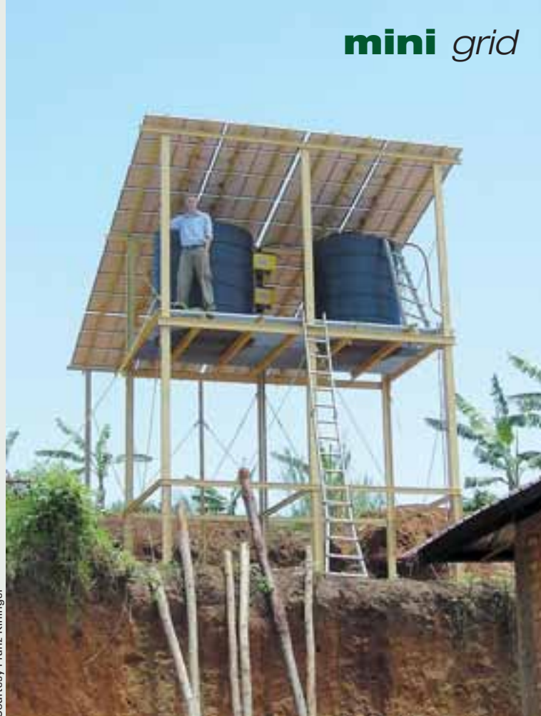
The author on the completed PV array, with the Sunny Boy, batteryless inverters visible in background. This array is 75 feet (23 m) from the battery bank.
