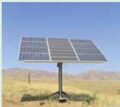
Left: The 1,000 W PV array. Right: The Whisper wind generator.
