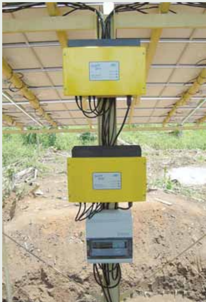
A close-up of the SMA Sunny Boy inverters and a junction box that combines their AC output.
