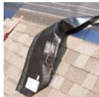
Below: Wiring leads on the back of a PV shingle.
