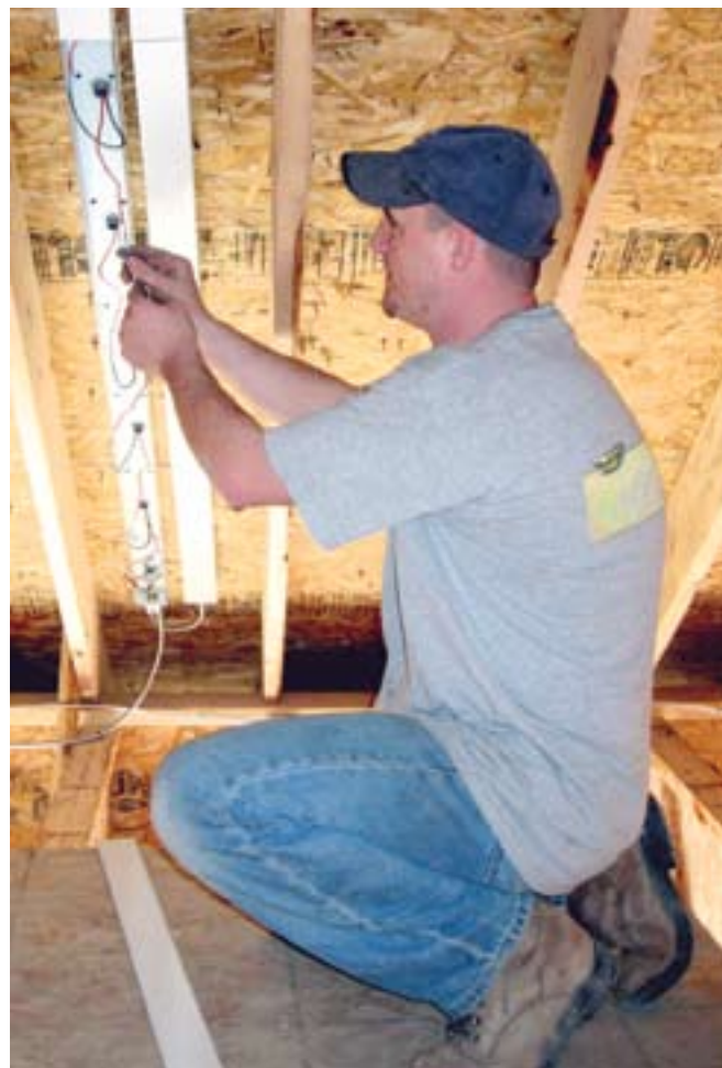
Making series connections in the raceway.
