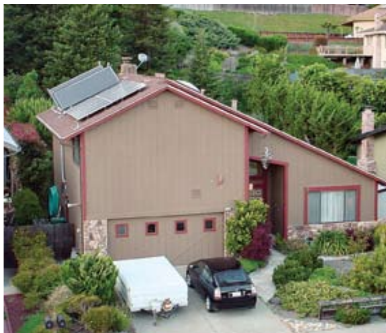
Two 4- by 10-foot thermal collectors (behind PV array) face due south on a west-facing roof.
