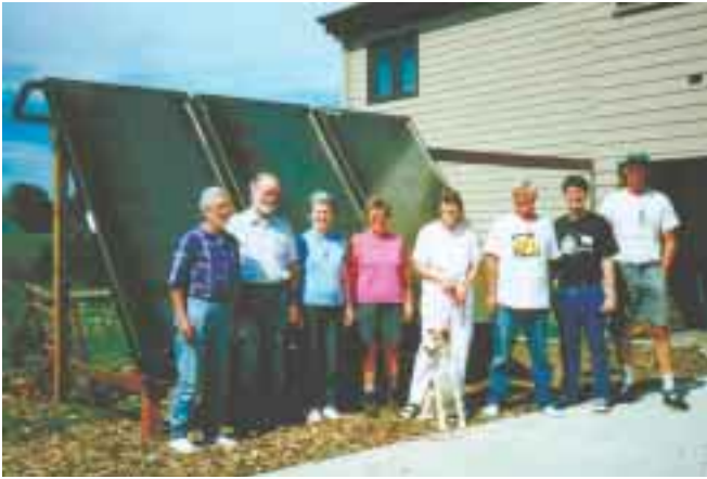
Solar Domestic Hot Water (SDHW) workshop at the Prairiewoods' guest house. Three of the Franciscan nuns participated in the workshop.
