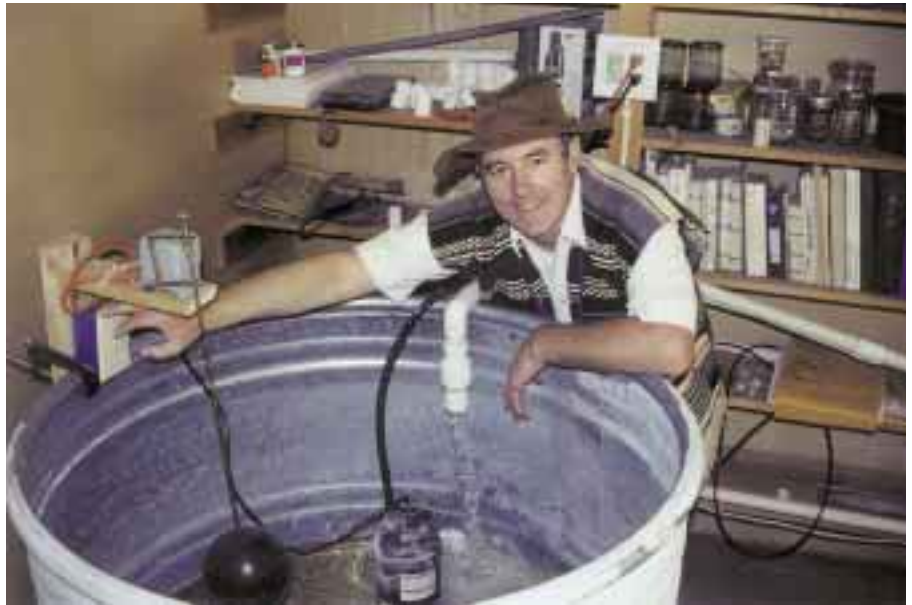
The AC well pump moves water to this tank. A sump pump pressurizes the irrigation water for distribution.
