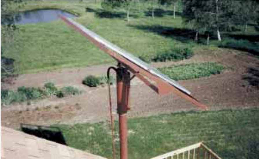
The PVs' top-of-pole mount eliminated the potentially dangerous roof mount.
