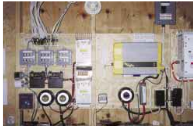
The Roll's C60 system with PROsine 1,800 watt and Trace PS2512 (off to right) inverters.
