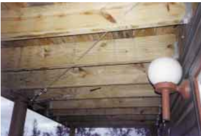
The tall pole is steadied just below the deck with cables.
