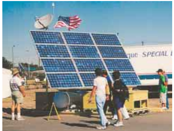
The Sacred Power 1.2 KW PV system that powered the exhibitors tent and stage.
