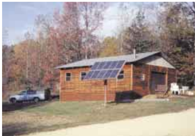
PV is portable! The upgraded system at its off-grid location in Tennessee.
