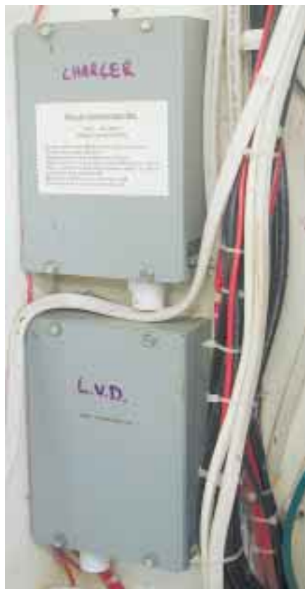
The voltage sensors and controls for the low voltage disconnect and AC battery charger.
