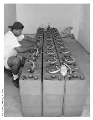
Solar electric systems can run on ordinary car batteries, but not for long. Car batteries are not designed for deep discharging drawing off lots of power. They're designed to crank out tons of amps to start a car, but they're the rabbits of the battery world. What you need is a tortoise, a battery that can give you all it has for long periods of time. No sprinters need apply.
