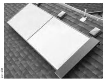
Fig. 3-3: The most prominent part of a solar hot water system is the solar collector. Collectors are typically mounted on the roofs of houses or alongside homes to ensure year-round exposure to the sun from 9 a.m. to 3 p.m. each day. Heat energy gathered from sunlight is stored in a water tank, usually located in the basement, for use when needed. This model by SolReliant uses a PV panel to provide electricity to pump. No additional wiring is necessary.
