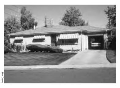
Fig. 6-6: Awnings can dramatically reduce heat gain through windows in the summer.
