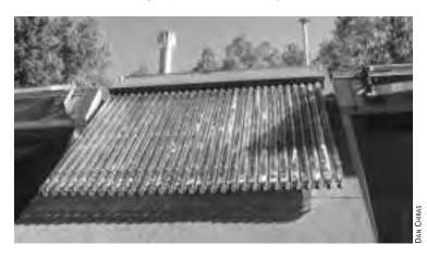
Fig. 1-2: Solar hot water panels like these convert solar energy into heat that is used to heat water for domestic uses and to heat homes. These glass tubes contain a small black copper pipe that is heated by the sun.
