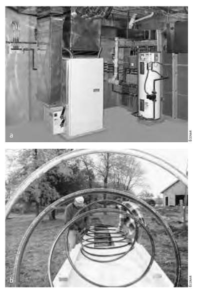
Fig. 2-8: Heat pumps like the one on the left in (a) strip heat from the ground via pipes (b) buried below the frost line.
