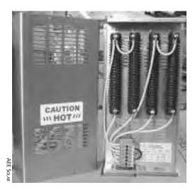
Fig. 9-11: Load diverters take excess energy and run it through resistors (shown on the right) to generate heat. They're useful in the winter to provide heat to living spaces as well as garages, sheds, and workshops.
