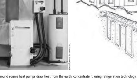
Fig. 4-11: Ground source heat pumps draw heat from the earth, concentrate it, using refrigeration technology, then pump the heat into the house. Pipes are laid horizontally in the ground 4 to 6 feet below the surface or vertically where they extend 100 to 400 feet below the surface. Water or a mixture of water and an environmentally benign antifreeze circulates through the pipe, gathering heat in the winter. A small electric pump provides the propulsive force.
