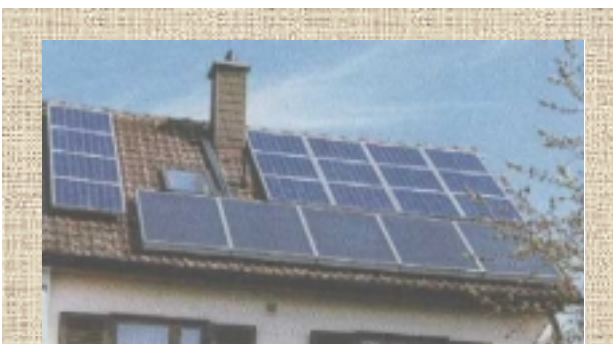
roof in Germany with 16 80-watt photovoltaic panels, which will generate around 1000kWhours of electricity per year – about one third of a family's needs. There are also 5 solar hot water panels at the bottom of the roof, which do not produce electricity – water passes through them and is heated directly.
