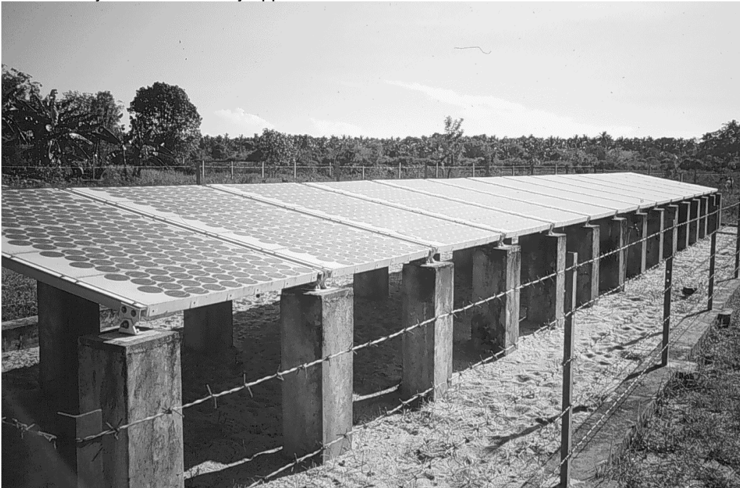
Figure 1: Array of PV Panels ©Smail Khennas/ITDG
