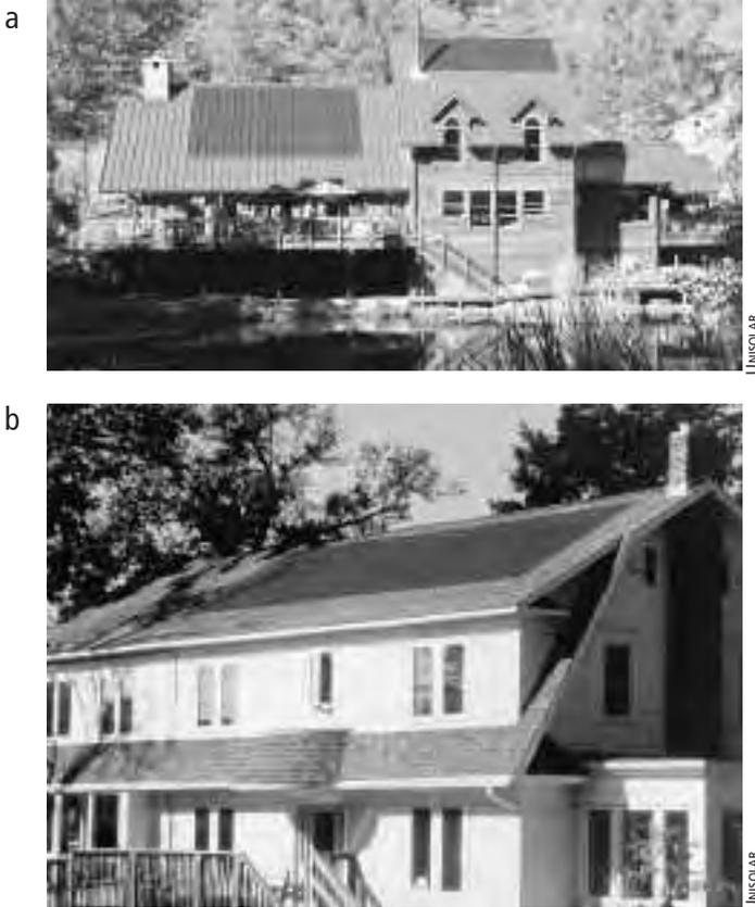
Fig. 7-12: Solar Roofing. Amorphous silicon ribbons can be used to make (a) long rolls of material that can be applied to standing seam metal roofing and (b) solar shingles. Both are forms of building-integrated photovoltaics.
