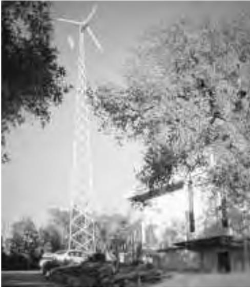
Fig. 8-8: The lattice or truss tower is strong and durable and an excellent choice for mounting larger wind machines. It can be supported by guy wires, if necessary.
