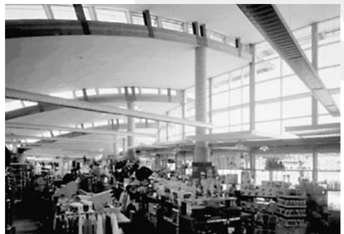
Fig. 12a, b: The Real Goods Solar Living Center, a retail store in Hopland, California, USA (designed by Van der Ryn Architects). A complete “bioclimatic” design, the building features passive solar heating, daylighting, natural ventilation and cooling, PV electricity and native landscaping. Energy savings compared to a conventional design in the Hopland climate are 90 %. In-store sales are 50 % higher than projected because the interior daylighting and comfort are so good.
