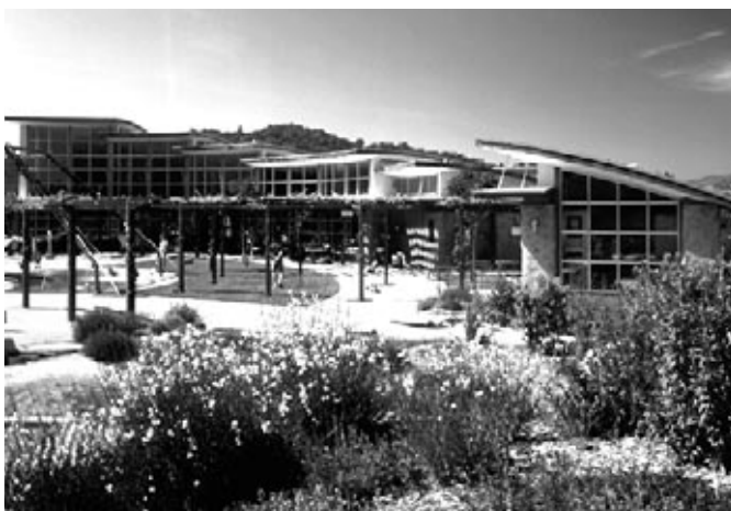
Fig. 12a, b: The Real Goods Solar Living Center, a retail store in Hopland, California, USA (designed by Van der Ryn Architects). A complete “bioclimatic” design, the building features passive solar heating, daylighting, natural ventilation and cooling, PV electricity and native landscaping. Energy savings compared to a conventional design in the Hopland climate are 90 %. In-store sales are 50 % higher than projected because the interior daylighting and comfort are so good.
