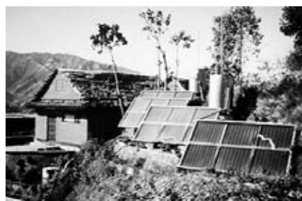
Fig. 13b: Solar water and space heating in Kathmandu, Nepal. Photograph by Dr. Donald Aitken
