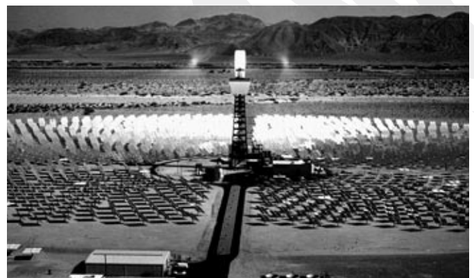
Fig. 14b: Solar I, the 10MW “power tower” in southern California.
