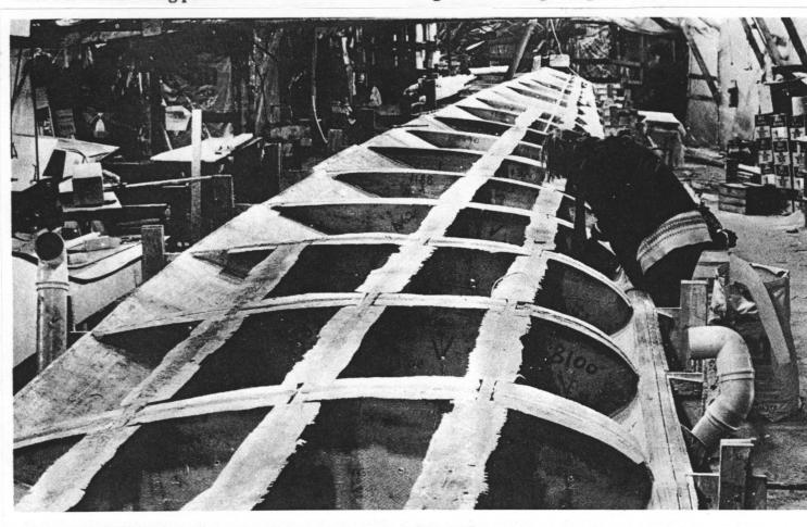
Wing-Sections with sawn-out "Flamingo"- Polystyrol blocks.
