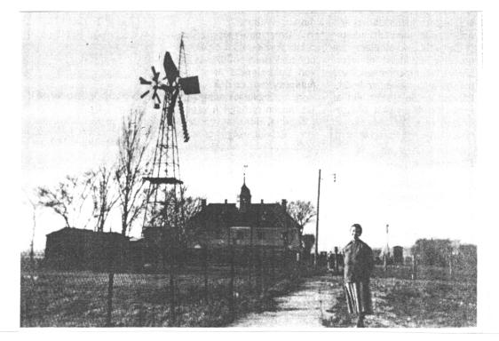
Wind-turbine of Type 1 - 1.5 built 1904. 10 kW DC Generator Tower height 17 m. Blade diameter 16 m. Sited in Copenhagen Harbour, in operation until 1957. This was a combined wind-turbine - petroleum spark ignition motor generator. Agricco wind turbine - designed by Vinding and Jensen - Denmark 1918 5 - 12.5 meter rotor-diameter. 40 kW asynchronous induction generator In production from 1918 - 1926. For further details:
