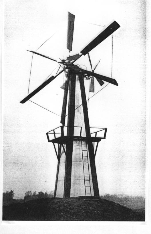
Modern re-construction of Type 0, for electrical power generation. Wooden blades, radius 4 m. La Cour-type Windmill for Electricty Production: Lykkegård model Denmark 1928.
