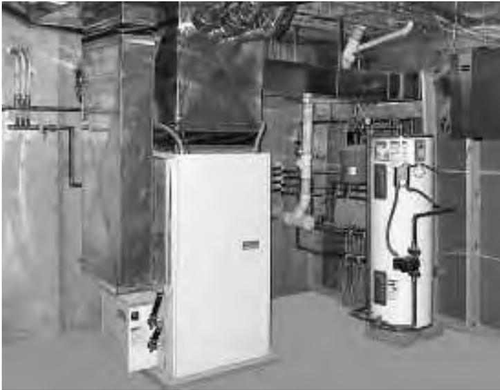
tank, the cold water cools the water in the storage tank. When the temperature of the water in the tank drops below the desired setting, the gas burner ignites in a gas-fired water heater. Once the water reaches the desired setting, the flame turns off.
