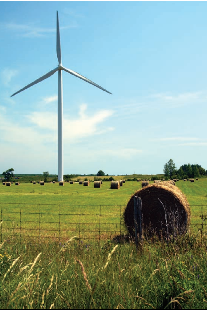
The tall tower and blades of a modern wind turbine. This turbine has a horizontal axis design.
