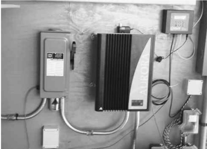
Fig. 8.1: *Grid-Connected Inverter.* This inverter by Magnetek is designed for batteryless grid-connected PV systems.
