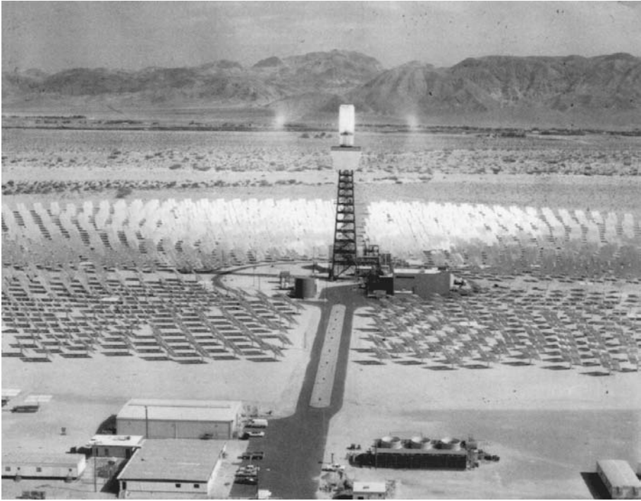
FIGURE 9-3 Solar II plant site view. (Source: U.S. Department of Energy.)
