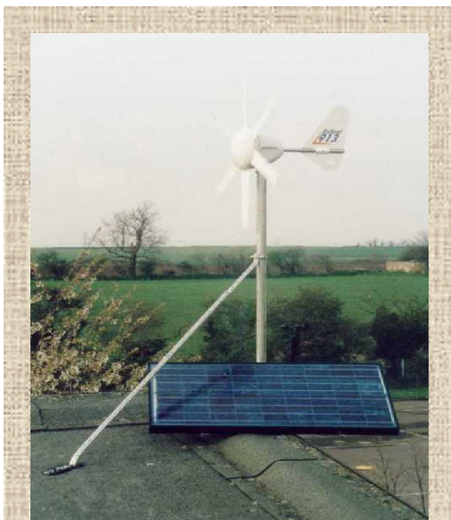
wind generators work well in combination with photovoltaics; solar provides more energy in summer, wind more in winter.
