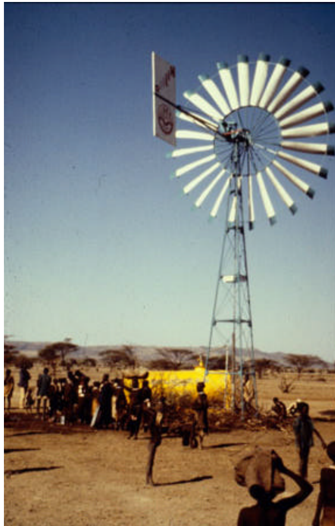
Figure 3: The Kitjito Windpump. Used to pump ground water in the Bhel region of Turkana for the Nomadic Pastorlists ©ITDG
