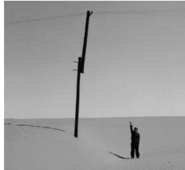
After more sand storms, the accumulating sand is carried to another location, leaving the extended pole far above the lowered land surface. Photo: Lu Tongjing.
