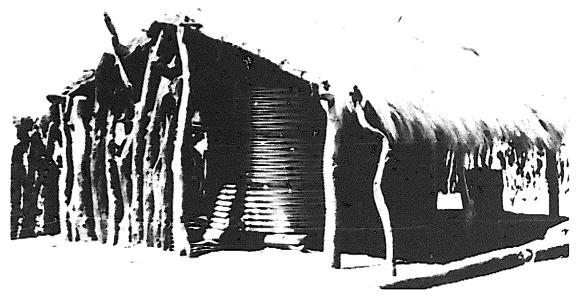
1-2 tonne metal grain tank, Swaziland, The tank is raised above ground to prevent bottom corrosion and shaded to minimize moisture migration. (Crown copyright, Courtesy TPI)
