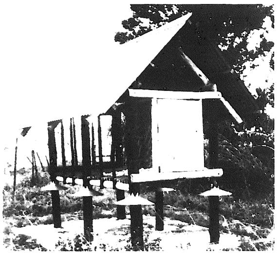
FPi ommended mesh-sided crib. Swaziland. Note the corrugated iron root and metal rat guards. (Crown copyright, Courtesy TPD)
