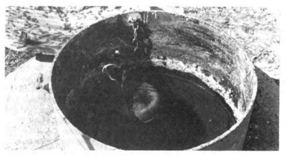
Float-valve regulates water level in stock tank.
