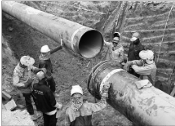
Building the Chad-Cameroon pipeline
