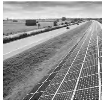
Solar panels as highway noise barrier, Freising
