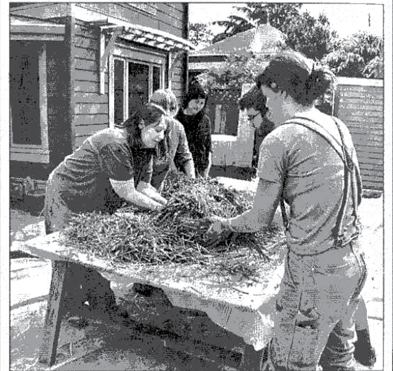
VBC volunteers knead straw with wet clay to pack as filler into the walls of a new teahouse, which will provide dense insulation. Photo by Carol Krause
