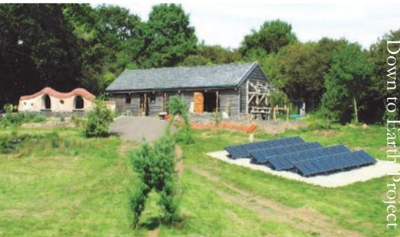
*The oak-tiled timber-framed building at Down to Earth Project, cob wall and 28KW solar array*
